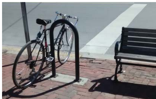
NARROW BASE HOOP RACK INSTALLED TOO CLOSE TO BENCH AND U-CHANNEL IN BRICK ON CARROLL AVENUE (SURFACE MOUNT ON CONCRETE BASE).
