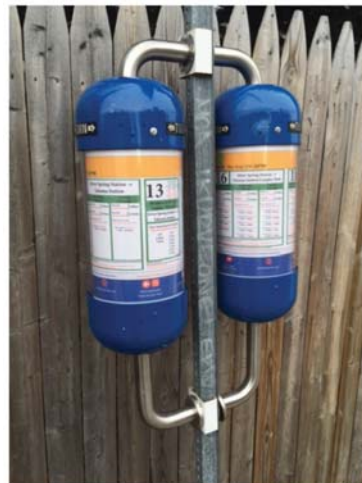
DOUBLE-TUBE AT PHILADELPHIA AND CARROLL AVENUES. NOTE SPECIAL U-CHANNEL ADAPTER.
